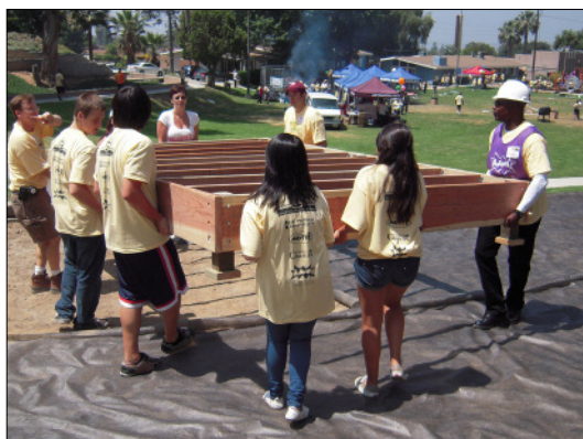
Volunteers lift part of a newly constructed amphitheater stage into place
